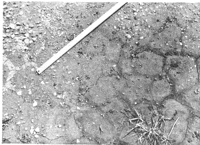
Fig. 3. Particles sorted into desiccation cracks near Fox River, Illinois. New cracks replace old ones, where particles are concentrated. The particles accumulated into the cracks increase from left to right, where more particles need sorting
