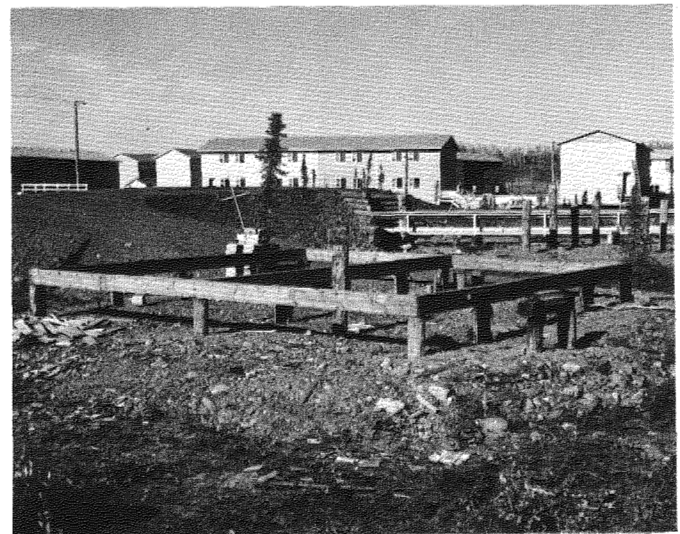
Fig. 4. Pile foundations for house.
