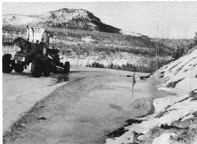
Fig. 7. Removal of ice from the road
