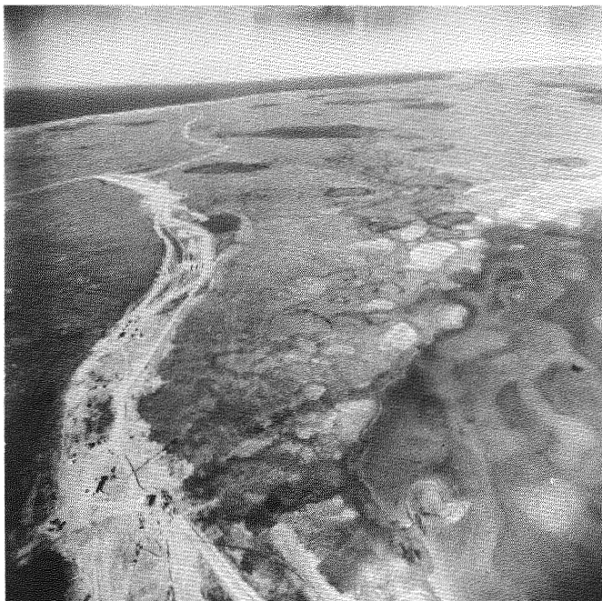
Fig. 7. Station in Foxe Basin. Note how layout of buildings, airstrip, and roads has been incorporated into the raised beaches. Level area to right of airstrip is entirely underlain by peat
