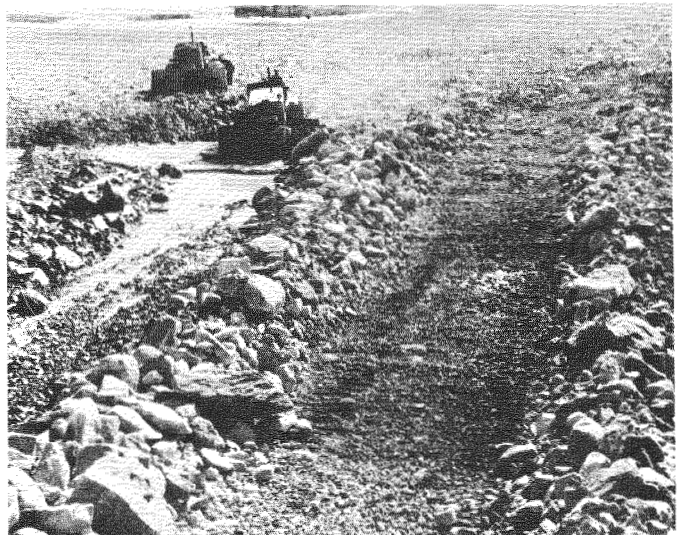
Fig. 2. Bulldozers stockpiling coarse fill from the active zone
