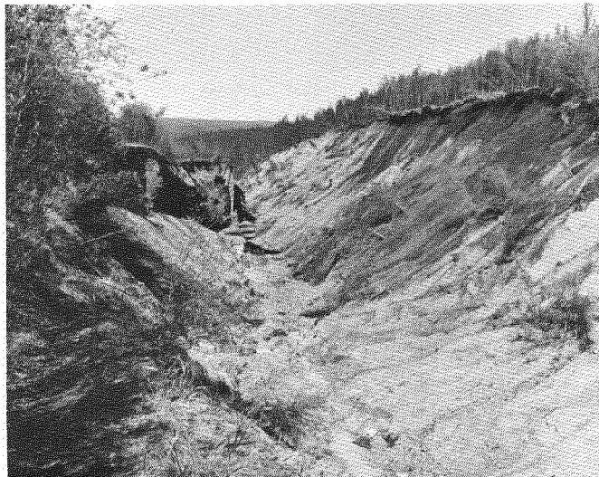
Fig. 7. View upstream in eroded spillway channel. Flat center area is at original elevation of the spillway apron
